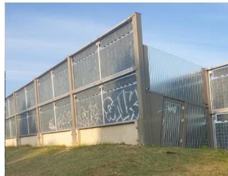
Another risk is vandalism. Unfortunately, attempts have been made to damage the barrier by throwing objects at it. This has led to a number of broken glass plates. Research has shown that this does lead to a dangerous situation. Also, it did not lead to a lower energy yield.
